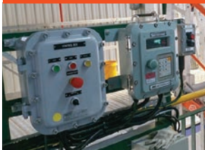
17 GROUNDING SYSTEM FOR TRUCK AND RAILCAR
