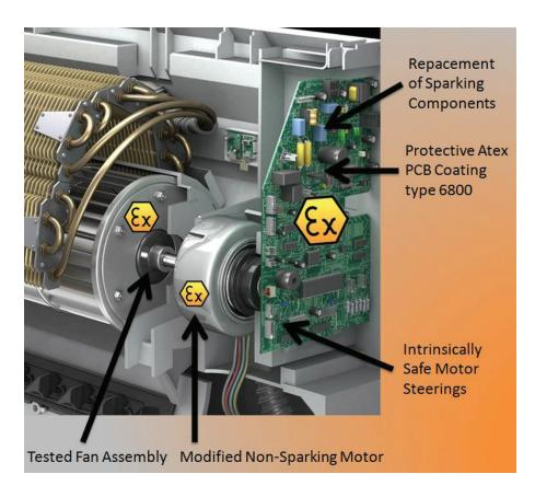
The above picture demonstrates some of the protective anti-explosion measures intergraded in Atexxo's indoor unit. All modifications are according to safety standards, well documented and tested. Standard units are available from Daikin, other brands can be delivered on request.
