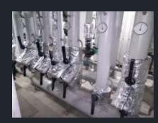
These are high quality products, designed and tailored by our lab and usable almost anywhere because modular for stratification depending on the temperature to be isolated and based on the conditions they are subjected to: exterior, interior, liquid, water, fire, thermal oil
